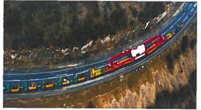
ASKI SİSTEM (GIRDER BRIDGE)
